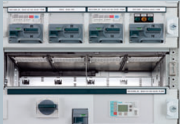
Miniature withdrawable adapter optionally with shutter
