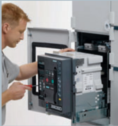
SENTRON 3WL in maintenance position: Inspection without circuit breaker removal
